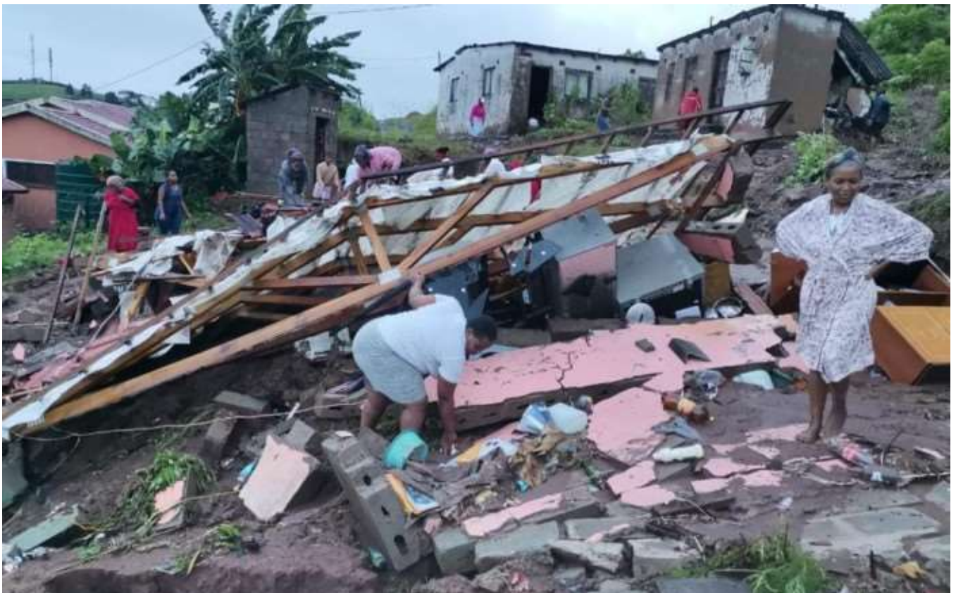
Catastrophic flood damage in KwaZulu Natal
